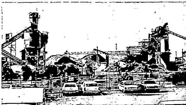
Extracting sand & gravel from the Salt River bed.
