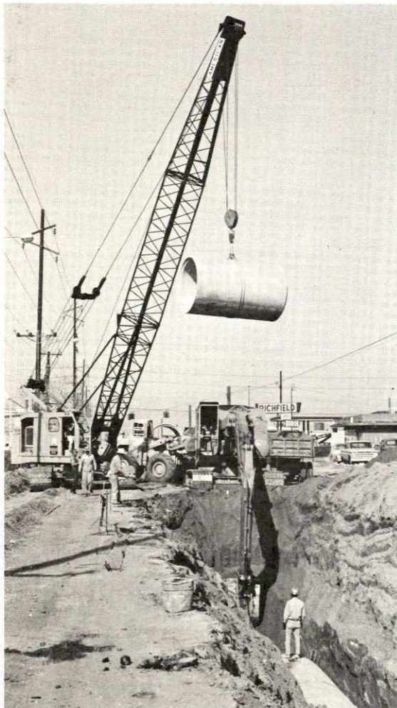
Storm drain installation
