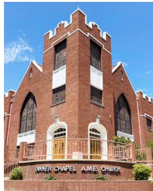
Tanner Chapel A.M.E. Church, listed on the Phoenix Historic Property Register in 2010
