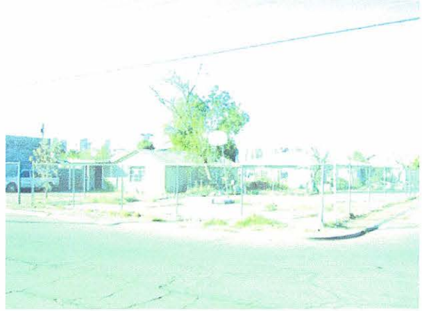
House demolition 1010 E. Hadley
