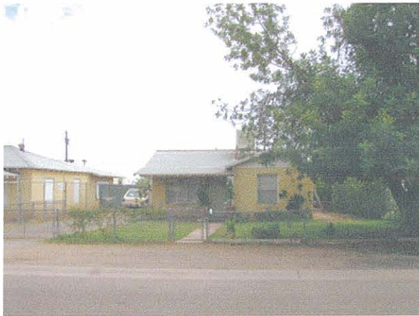
Front-gable-and-wing 3337 E. Jefferson Jesus Leyva House Built c. 1955
