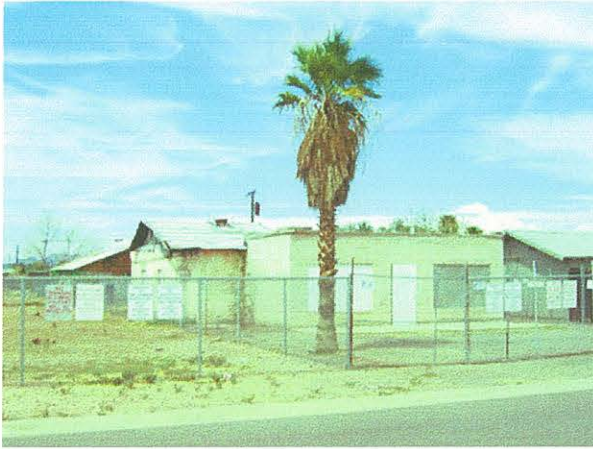
Inappropriate commercial conversion
