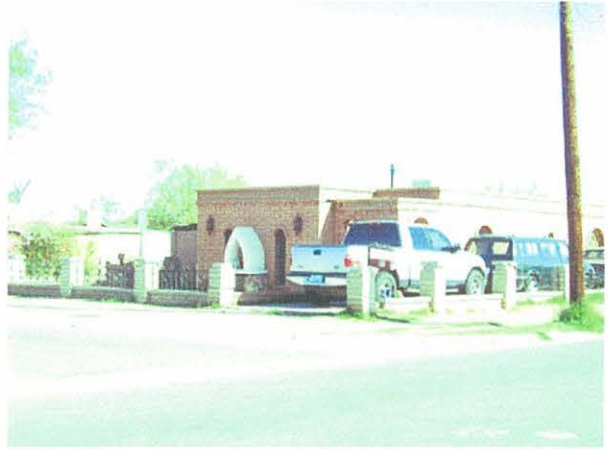
904 S. 10 th Street Slump block veneer applied during the modern era.
