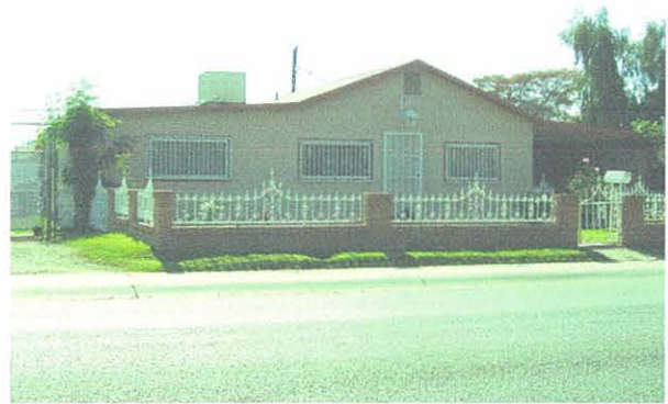
1305 E. Mohave Street Inappropriate stucco veneer and window treatments.
