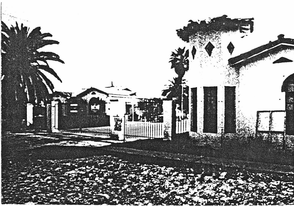
FIGURE 44 STRIP COMMERCIAL King's Rest Hotel Motor Court (63-8), (1984).
