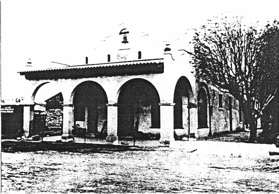
FIGURE 13 EARLY URBAN CENTER PERIOD Curio Store (c.1915), now demolished. Mission Revival Style. State Library and Archives.
