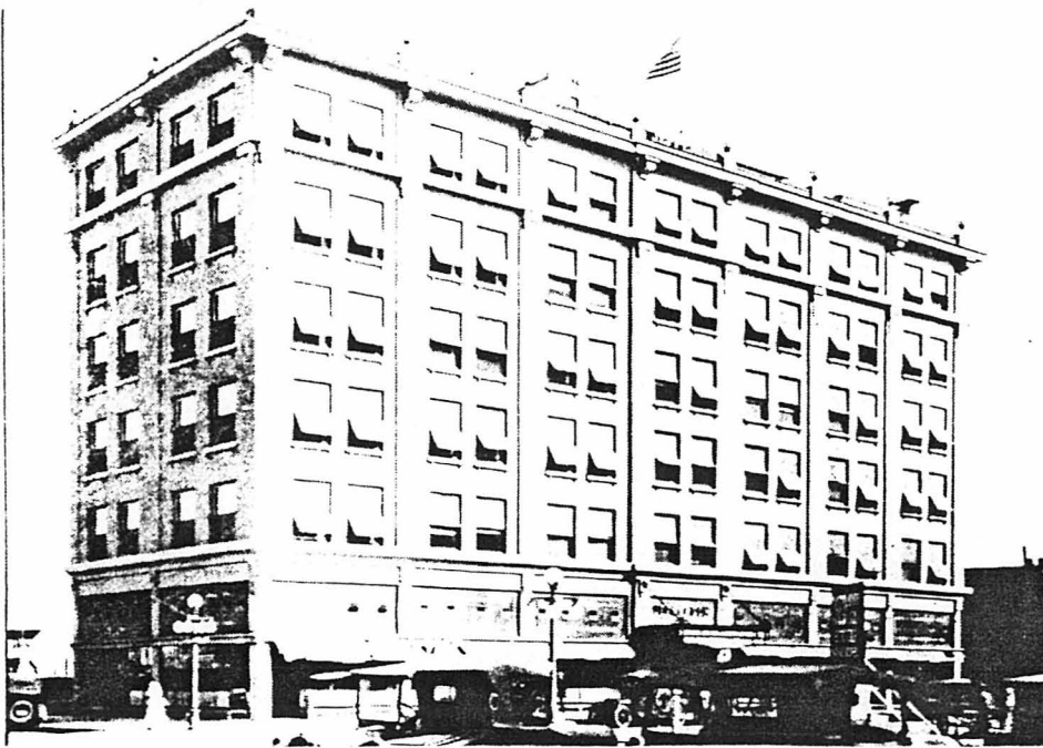
FIGURE 14 EARLY URBAN CENTER PERIOD Jefferson Hotel (Ackel Building), (30-5), (c.1915). State Library and Archives.
