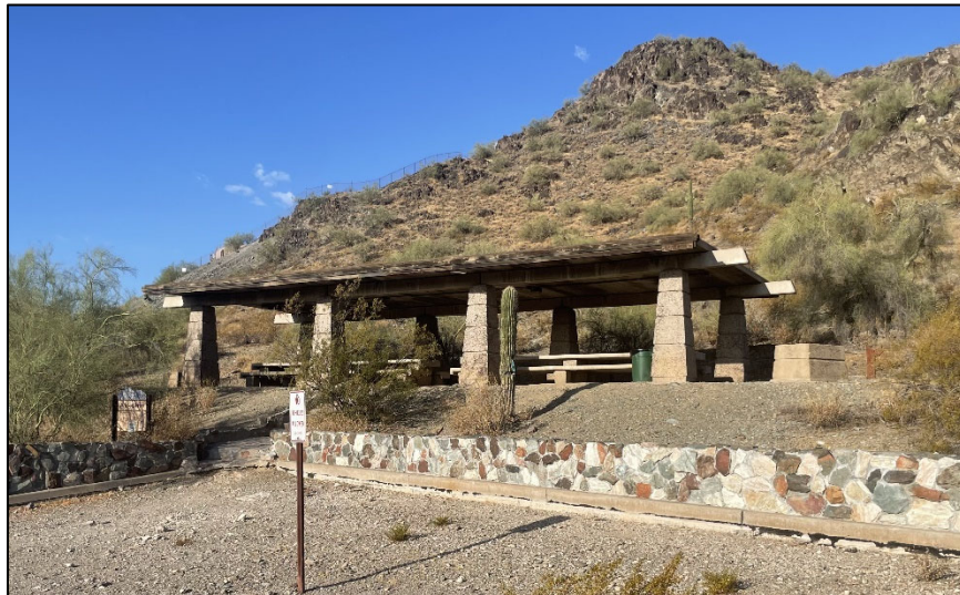
Figure 4. Overview of Ak-Chin Ramada (Building 3D), view facing southwest. The retaining walls appear to be modern (post 1974).
