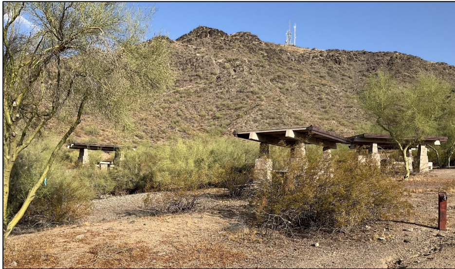
Figure 5. Overview of smaller ramadas, each with a single table and barbecue pit (Buildings 3E-3K). View facing northwest.
