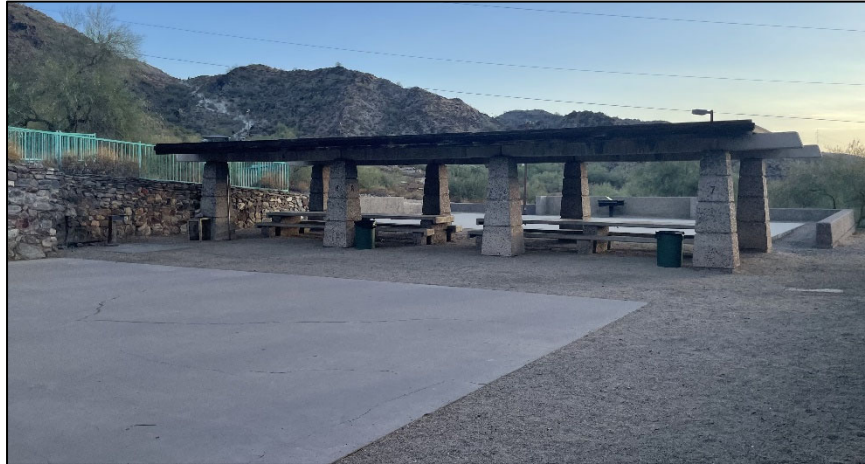
Figure 7. One of the ramadas of Building 2D that encompass the concrete event slab, surrounded by with wet-laid stone and concrete retaining walls. View facing northeast.
