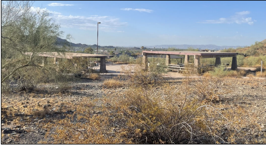
Figure 1. Overview of Yavapai Ramadas (Buildings 3A and 3B), surrounding a concrete event slab, view facing south.
