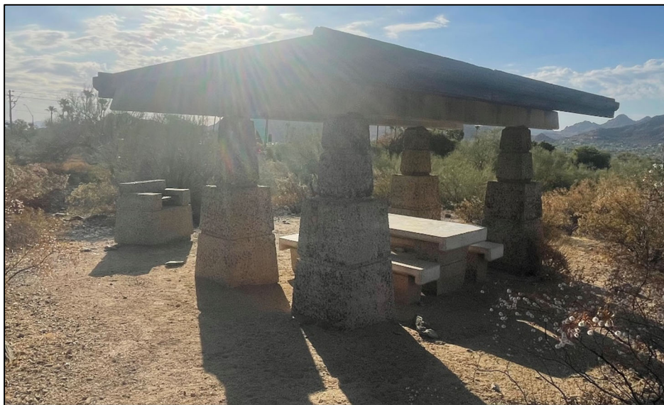
Figure 6. Overview of Building 3K, a small ramada table and barbecue. View facing southeast.
