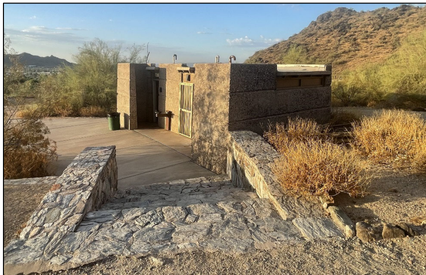
Figure 4. Overview of restroom facility (Building 2C) with modern stone retaining wall and steps, view facing south.
