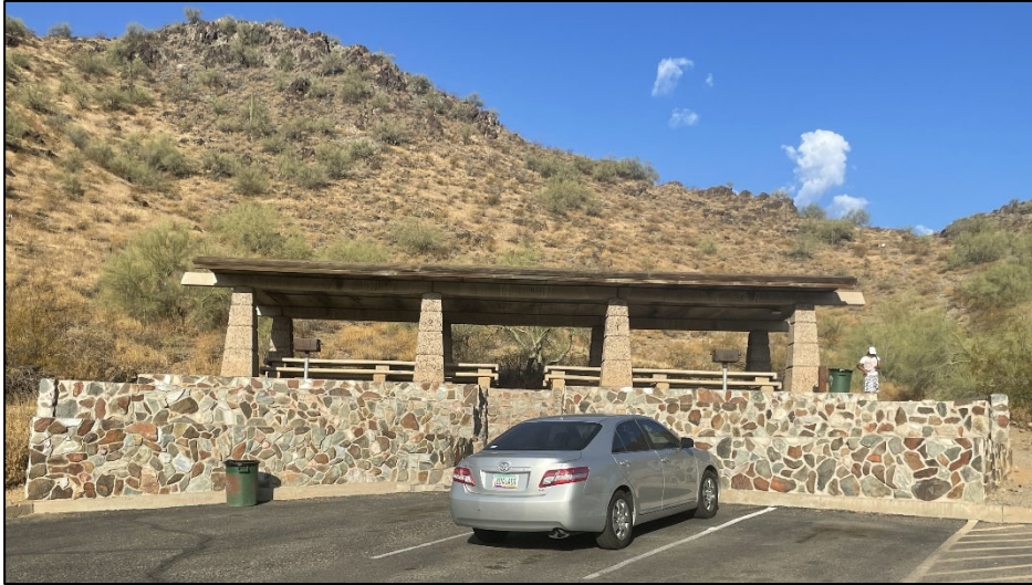
Figure 3. Overview of Quechan Ramada (Building 3C), view facing west.
