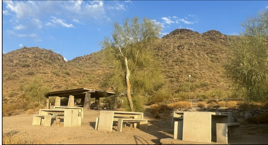
Figure 3. View of modern concrete tables with the unnamed ramada in background (Building 2B), view facing northwest.
