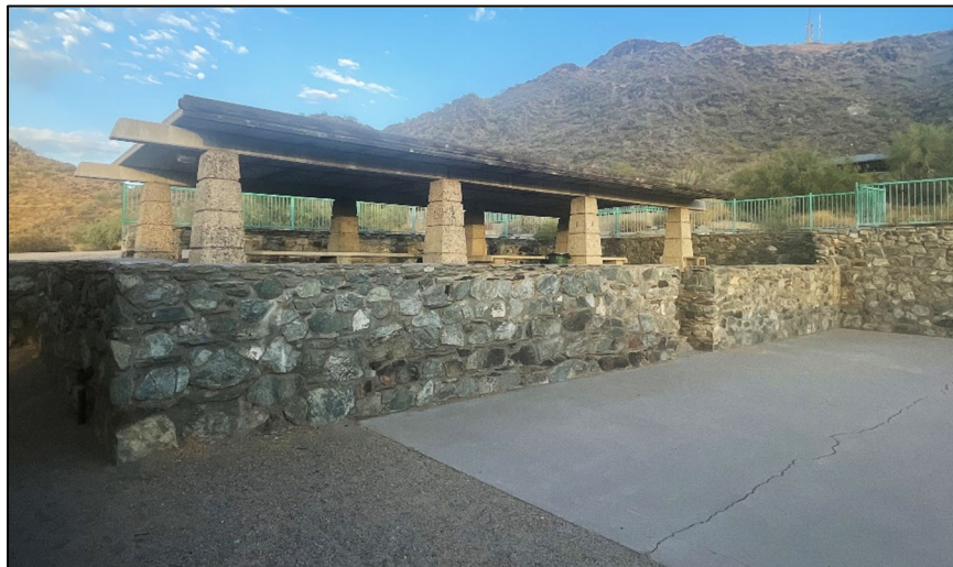
Figure 6. One of the ramadas that surround the concrete event slab in Building 2D. The placement of ramadas and perimeter retaining walls (wet-laid stone and/or concrete) effectively forms a recreation courtyard. View facing west.
