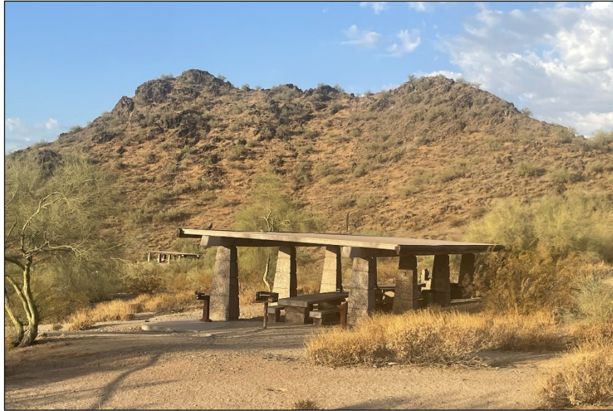
Figure 2. Overview of the park and natural setting from Building Group 2, view facing south-southwest.
