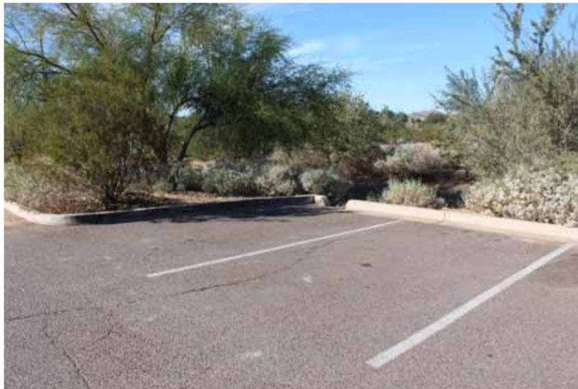
**Photo 46.** Parking curb cut for drainage. View to northwest. Photograph taken on November 18, 2014.
