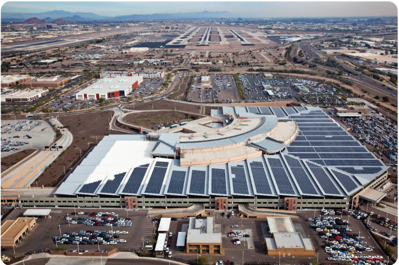
Solar Energy Generation System at Rental Car Center at the Phoenix Sky Harbor International Airport
