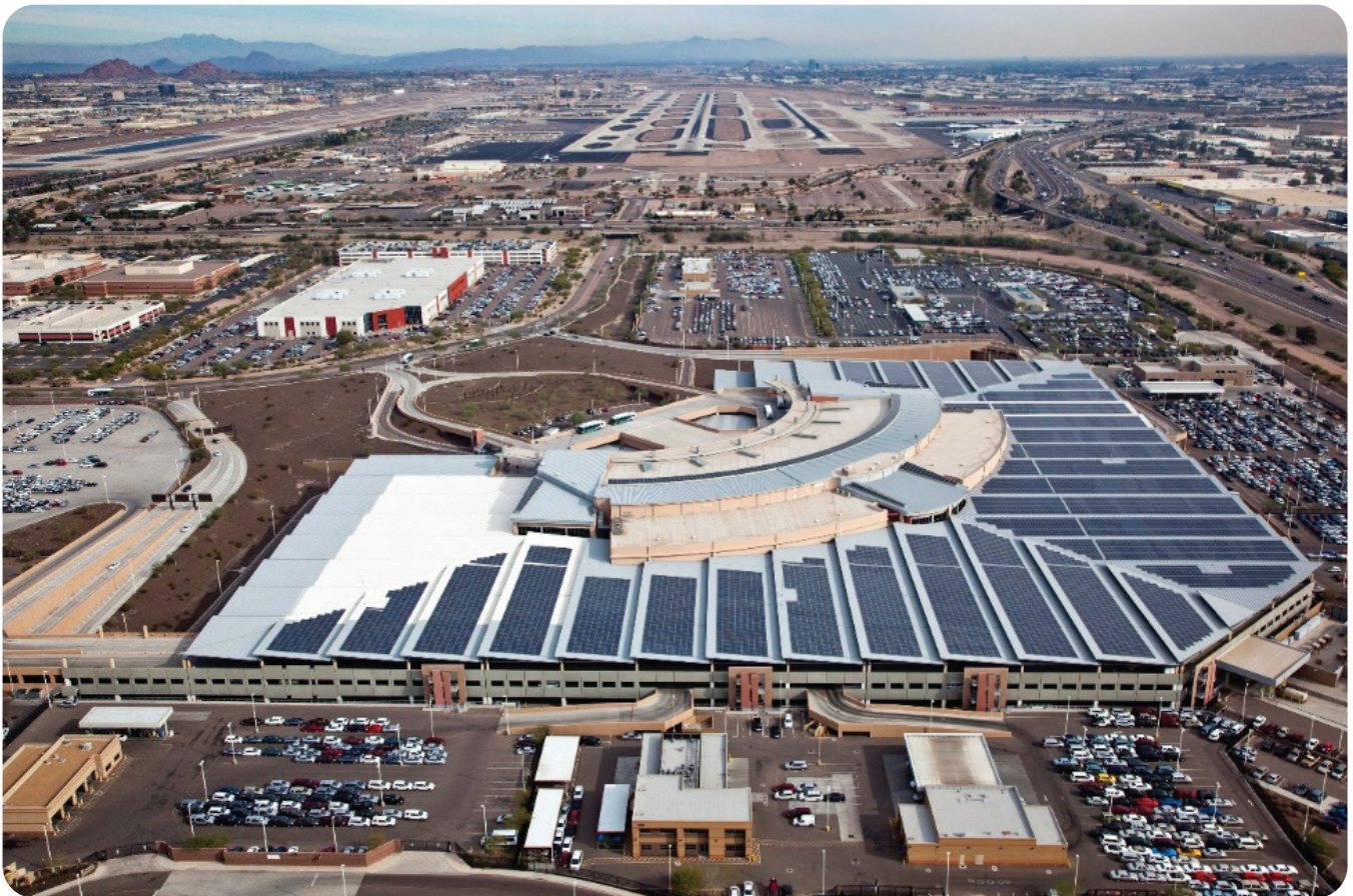
Solar Energy Generation System at Rental Car Center at Phoenix Sky Harbor International Airport
