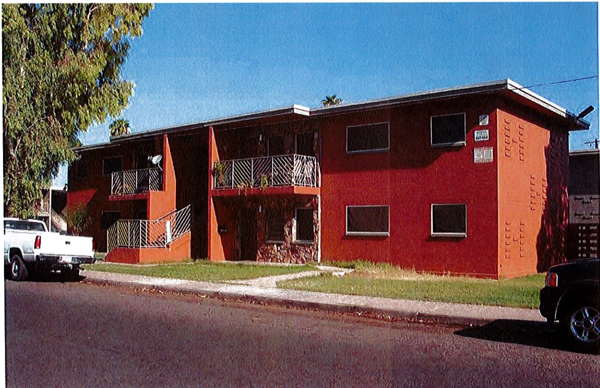
A.L. Krohn AZ 1-8B building with stone veneer and patterned block (EcoPlan Associates, Inc. 2012)
