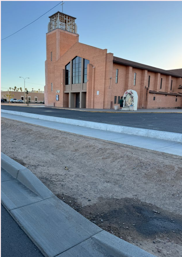
Project: Central Ave. project under construction
